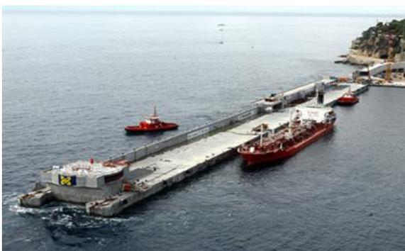
Fig.1 Floating breakwater in Condamine
