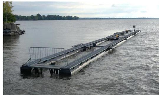
Fig.7 Floating breakwater of port Tiffany Wharf
