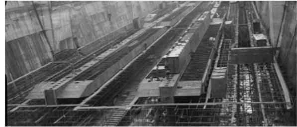
Fig.5 Construction of bombardon floating breakwater
