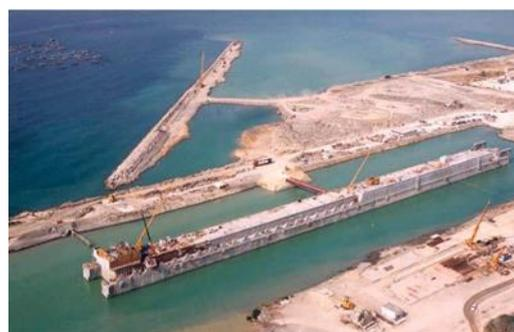
(a) Construction of floating breakwater in Morocco
