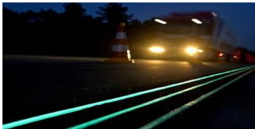
Fig-5: Glowing highway through photoluminescent
