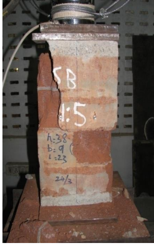
Fig. 5 Typical failure of CSEB masonry Prism, CM 1:5 in loading frame
