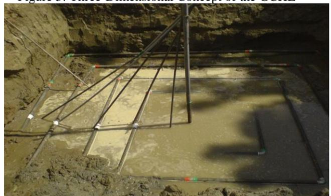
Figure 6: Final installation of GCHE before burying underground.
