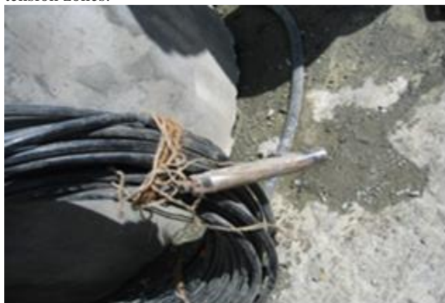
Fig. 9 Instrumentation of Tehri Dam 1
