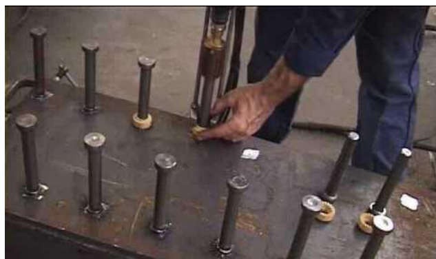
Figure 1. Shear connector
