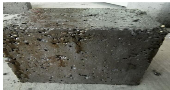
Fig.2. After demolition of the tested block
