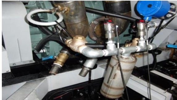
Fig. 4 Photo of Measuring Condition ②
