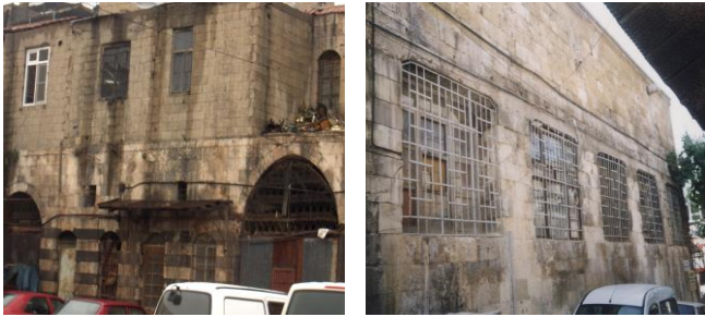
Figure 2. Examples of darkening - color change on the surface of a building
