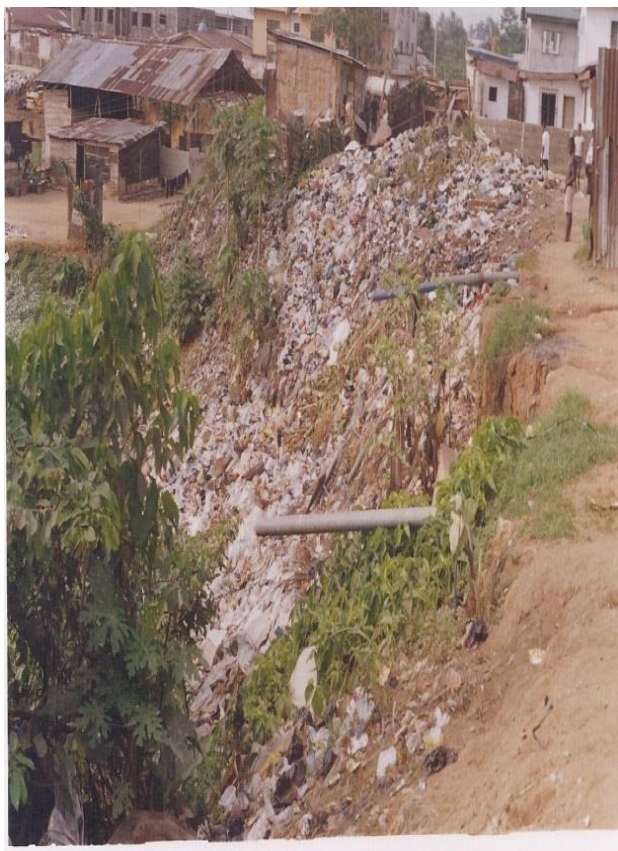
Plate 1: Municipal wastes dumped into the Borrow Pit (sewage pipes channeled directly into Borrow Pit)
