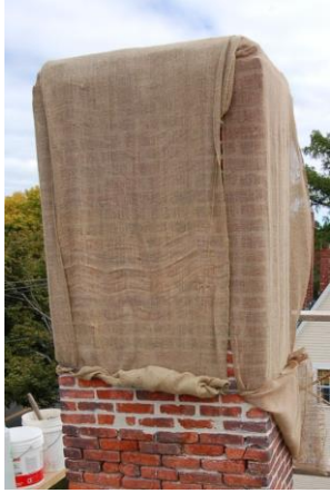
Curing of vertical member bricks
