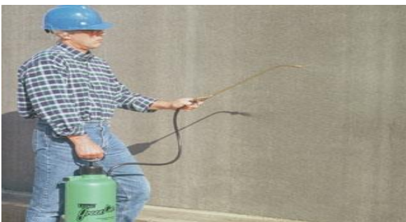
Curing using chemicals sprayed on concrete
