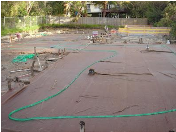
Curing of concrete slab using gunny bags
