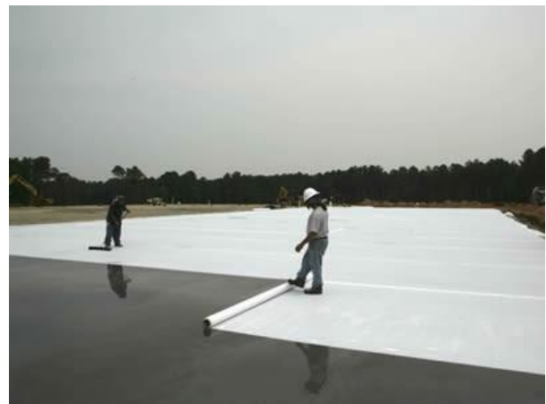
Curing of concrete slab with covering plastic
