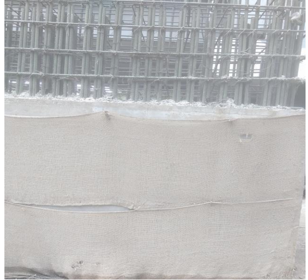
Curing of vertical member using gunny bags
