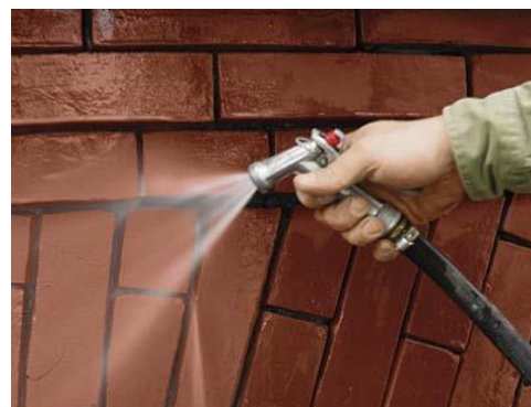
Spraying of water on bricks
