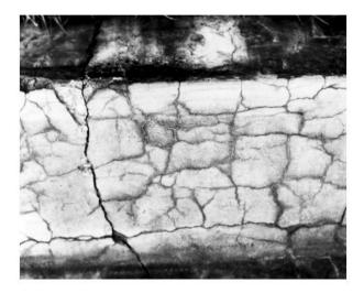
Fig 2: Photograph of typical surface map-cracking due to ACR (Ref. ACI 22.1R-98) [8]
