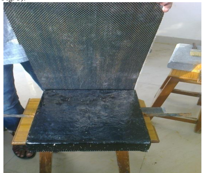
Fig. 2 Wrapping of FRP sheet after coating Epoxy paint
