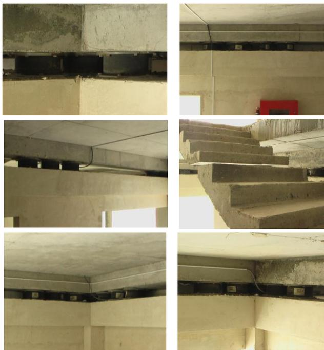
Fig. 5. Examples on installation of rubber bearings' clusters in the 17-story base isolated apartment building "Sevak" in the course of construction
